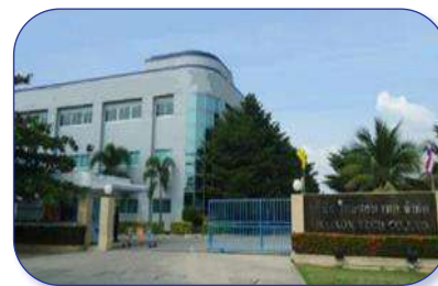
Plant 3 Thaixion Tech
